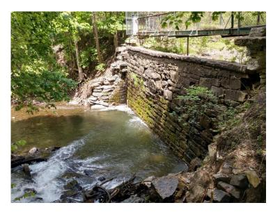
Approximately 10 years ago, DCR partnered with the City of Pittsfield to stabilize the sluiceway, and since then has annually cleared sluiceway debris in order to maintain the lowest feasible water level at the dam. In addition, ODS staff periodically inspect Bel Air Dam as part of regular patrols to identify issues and implement minor repairs and maintenance as needed.
